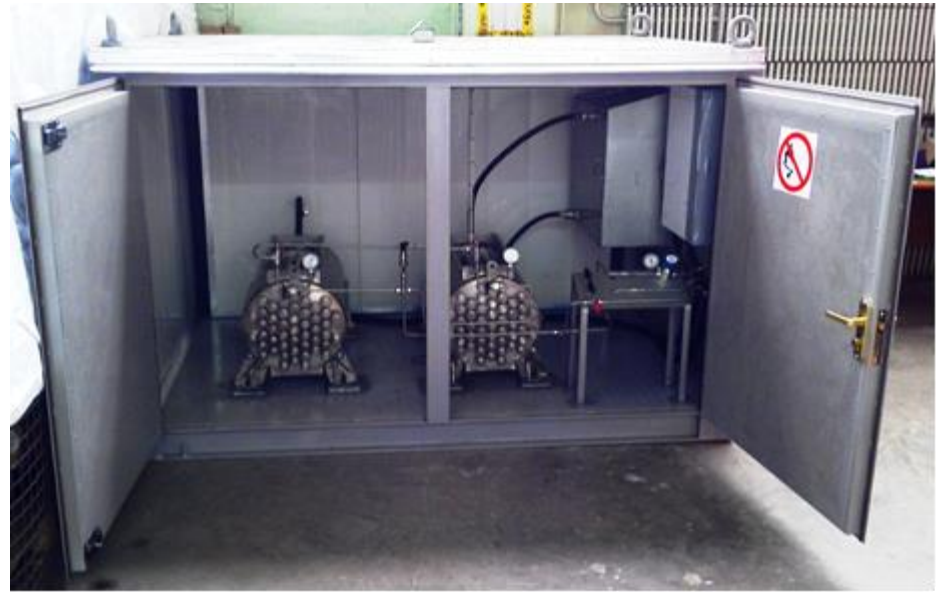
25 kWh metal hydride storage for 10 kW PEM FC renewable energy system
