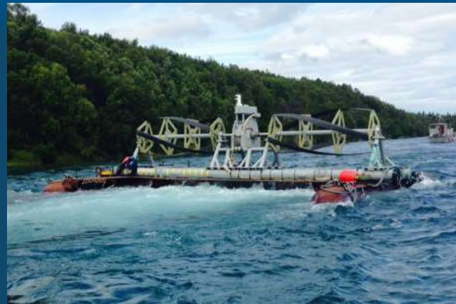
There were 3 hydrokinetic turbines installed in Alaska this summer, including the community of Igiugig (above)
