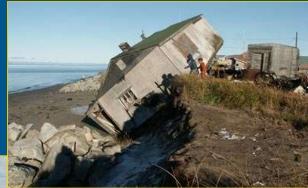
Erosion from fall storms - Shishmaref
