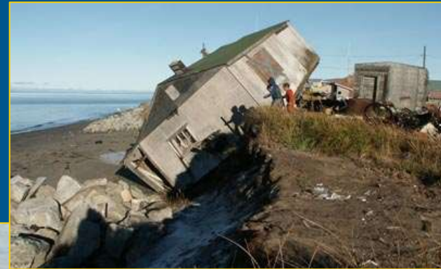
Erosion from fall storms - Shishmaref
