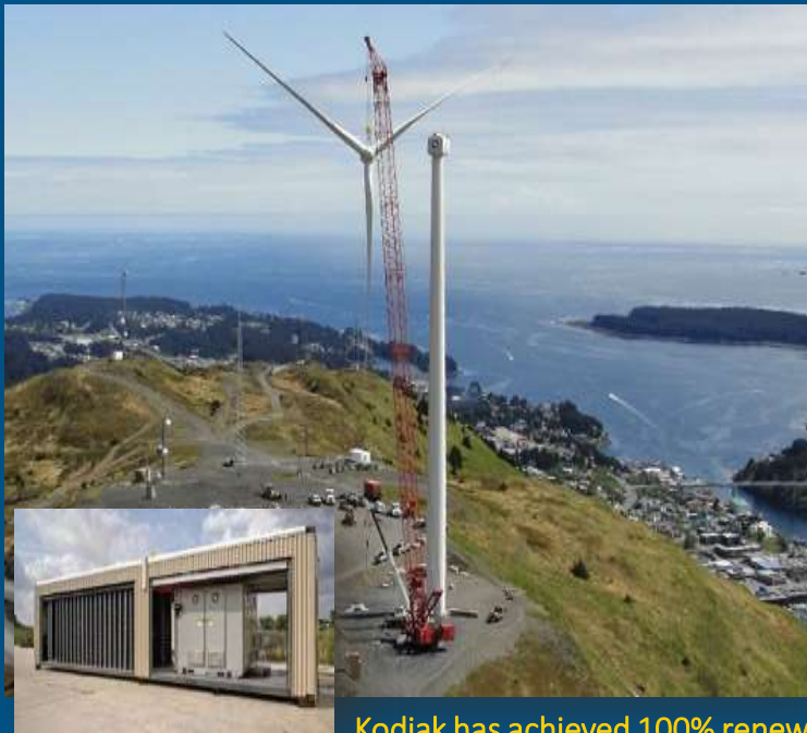
Kodiak has achieved 100% renewable penetration with hydro-wind-battery-flywheel system (above)
